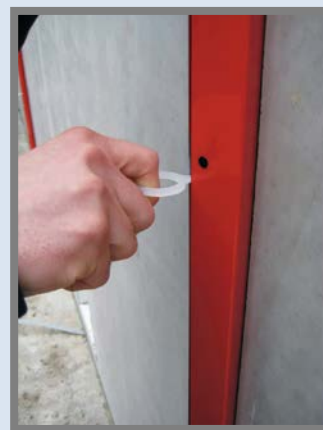
3. Rotate and drag FLUXX anchor for fixing the rail FLUXX
