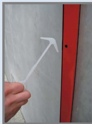
2. Inserting the FLUXX anchor through the opening of the FLUXX rail
