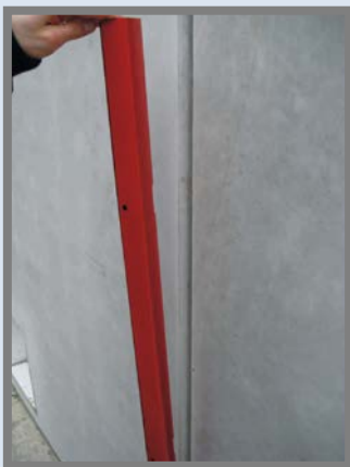
1. Creating the FLUXX rail at the butt joint to be sealed
