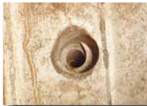
wire loop for M 24, SWL 35 kN
